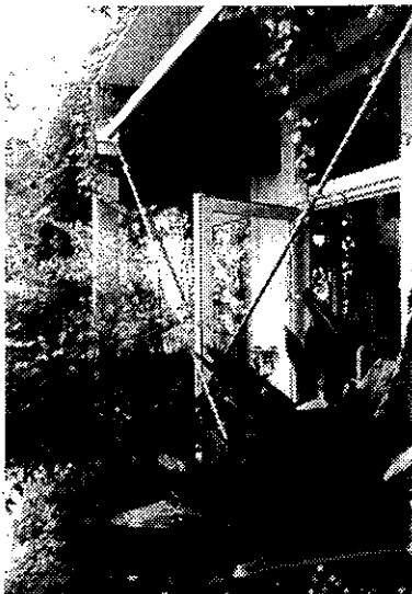
Figure 27: Lower office pavilion Photo: G. Löhnert
