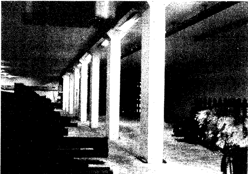
Figure 3: The open basement under the warehouse hall. In the background, one of the air outlets can be seen.
