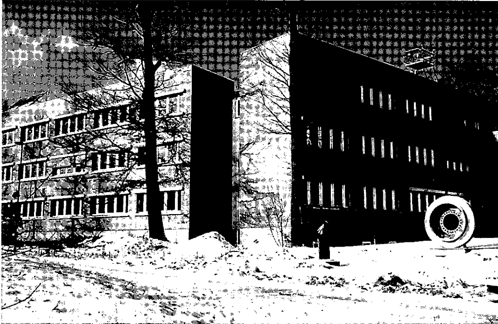
Fig. 1: A view of the ENTE-building from the south-east
